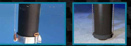
Add and splice vertical and horizontal nonmetallic reinforcement, if desired, while lowering the system in water.
