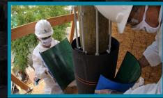
**4** Outer shells are added and bonded together with joints staggered to complete structural continuity in both hoop and vertical directions.
