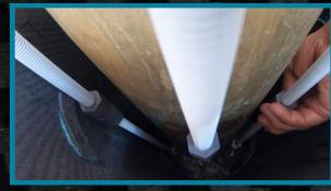
Pump polymer grout into the annular space around the pile from bottom up to complete process.
